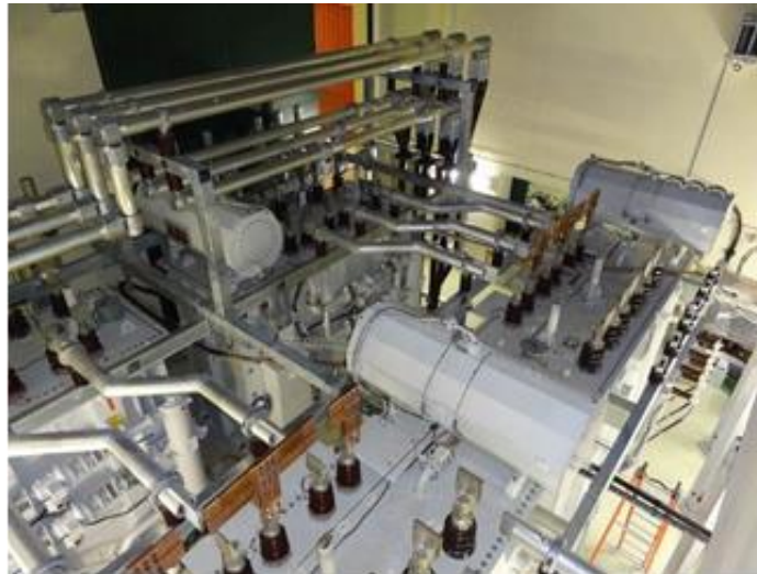
Figure 2. KWO Synthetic Ester Transformer Installation
